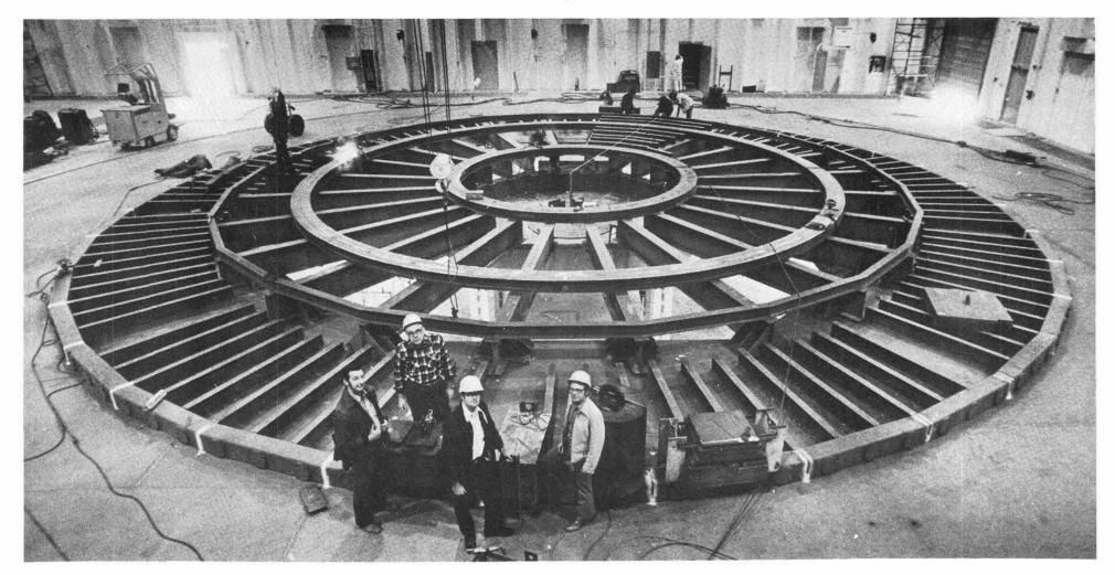
STEEL SUPPORT STRUCTURE for Sandia's EBFA-I (Electron Beam Fusion Accelerator) is shaping up in the new facility building south of Area I. Components of EBFA-I are being fabricated in machine shops throughout the state. Accelerator assembly should be complete and the experiment operational in June 1980. In the meantime, construction of a new office and laboratory building is nearing completion; occupancy by the staff of Fusion Research Department 4240 and Pulsed Power Systems
